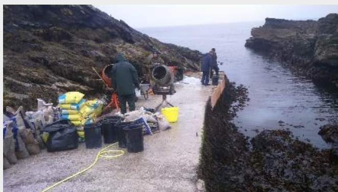
Slipway Maintenance – Aron Sapsford
