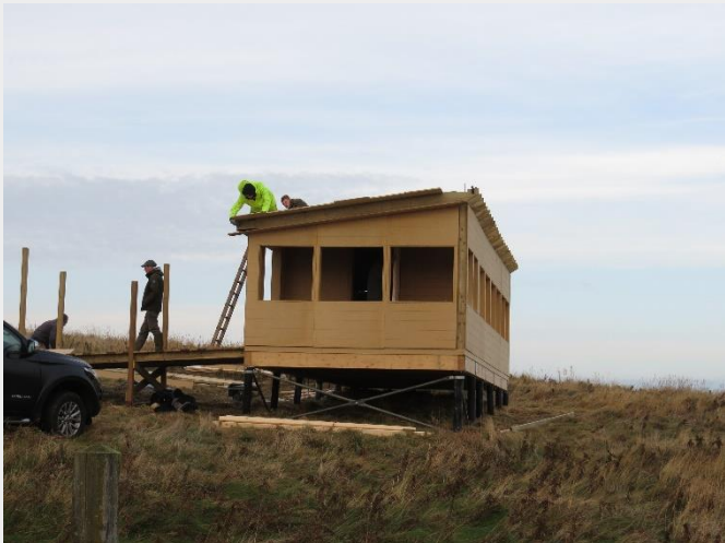
Construction of the seawatching hide – Craig Thomas
