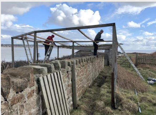
Trap repairs - Steve Williams
