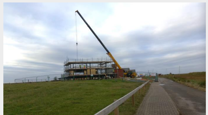
New Visitor Centre under construction – Jim Shaw
